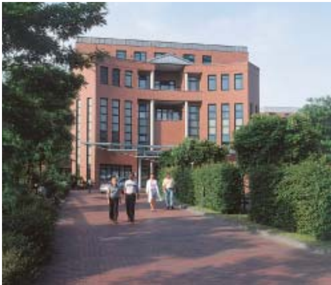
Main entrance Klinikum Oldenburg
